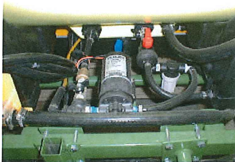
Figure 2: CDA filter shown next to red handled 3-way ball valve
